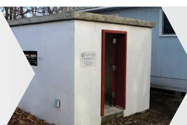
The ability in the design of a Fox Blocks safe room provides the resiliency to resist a combination of severe weather events – hurricanes, tornado, floods, and fires. The military has successfully tested and recognized ICFs for resistance to explosions. The properties of Fox Blocks do not promote mold or mildew growth and create a safe indoor air environment.
